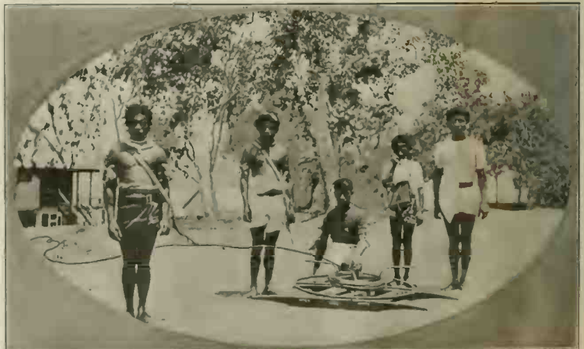
A Tropical Telephone Wiring Party, Composed of Native Boys, Who Work Three Years for Their Government At the Rate of $2.50 Per Month!
